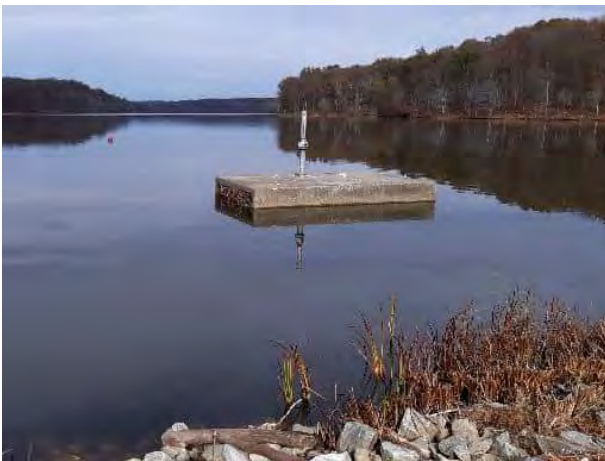
Above-water portion of riser
