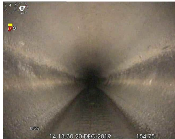
Conduit interior (typical)
