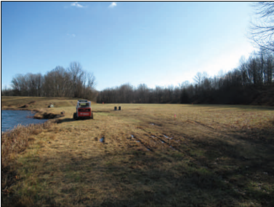
Figure 6-9. Emergency Spillway, Facing South
