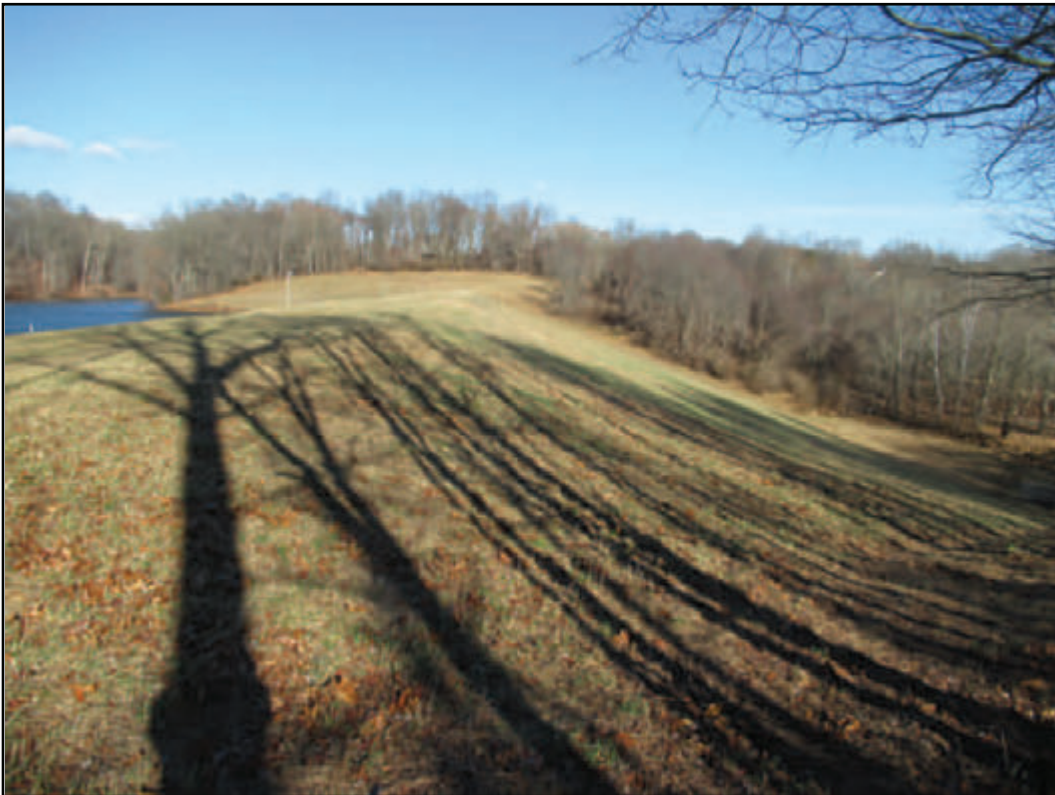
Figure 6-8. Piney Run Dam, Facing East
