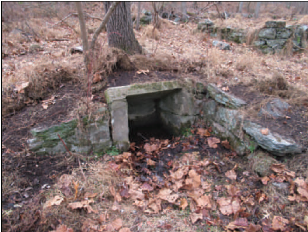
Figure 6-29. 18CR293, Feature 3, Facing Southwest
