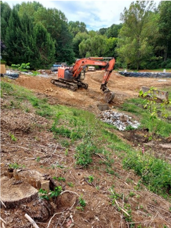
Construction is underway at the Saint George's Gate retrofit project.
